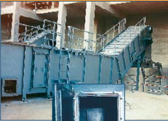
Inspection gate of an ash conveyor
